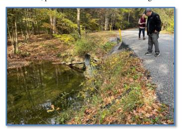
Ben then showed us a large, open culvert that is being installed on Wolf Den Run, a tributary of the North Branch of the Potomac. The culvert will be large enough and low enough to allow Brook Trout to move upstream and downstream, reconnecting
